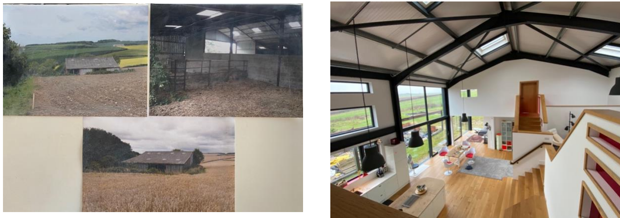
Fig.26 The Barn as it was (L) and as it is now (R) It has a sealed shell with ground source heat pump and mechanical ventilation
