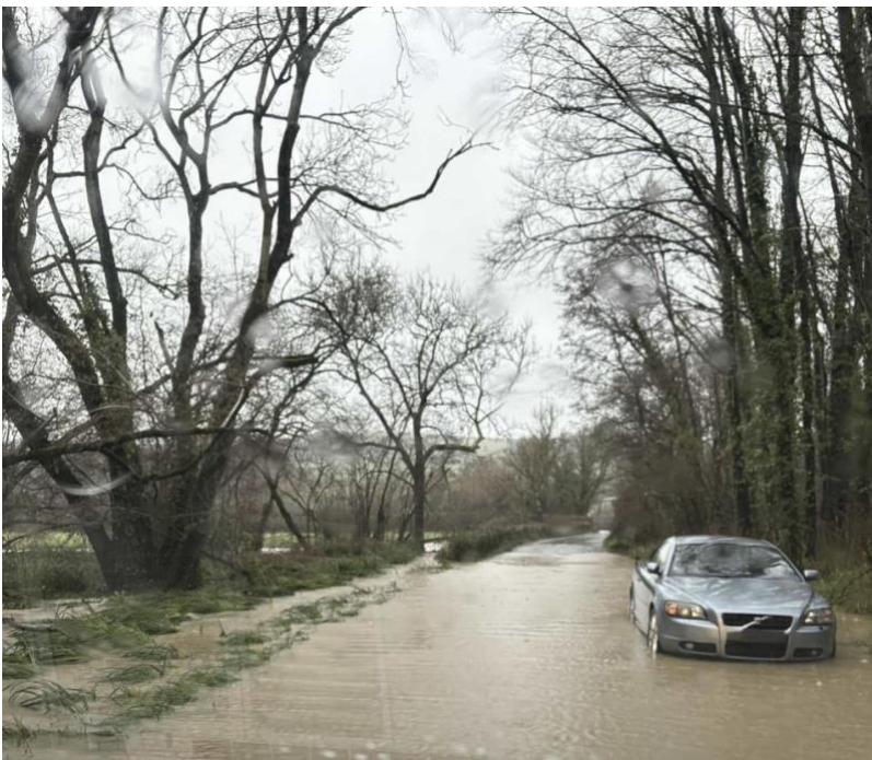
Figure 8 The Road at Chicks Bridge impassable to traffic in heavy rain.
